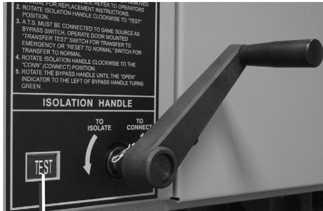
Figure 3-19. Isolation Handle turned to TEST .
