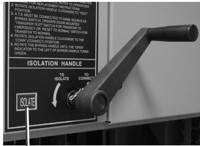
Figure 3-12. Isolation Handle turned to ISOLATE .
