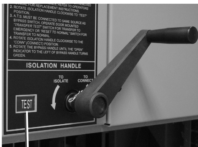
Figure 3-10. Isolation Handle turned to TEST .
