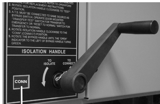
Figure 3-21. Isolation Handle turned to CONN .
