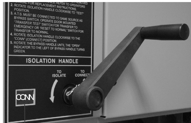
Figure 3-21. Isolation Handle turned to CONN .
