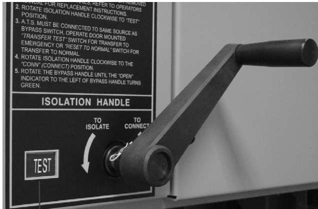
Figure 3-19. Isolation Handle turned to TEST .
