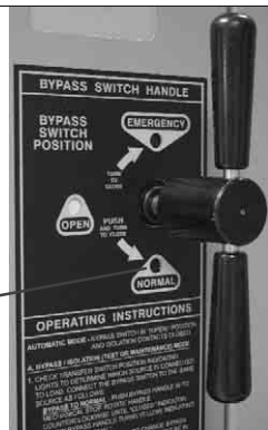
Figure 3-6. Status light and window indicator for Bypassed to Normal Source.
