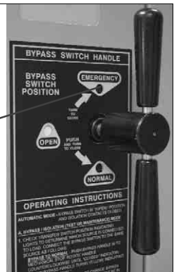
Figure 3-8. Status light and window indicator for Bypassed to Emergency Source.
