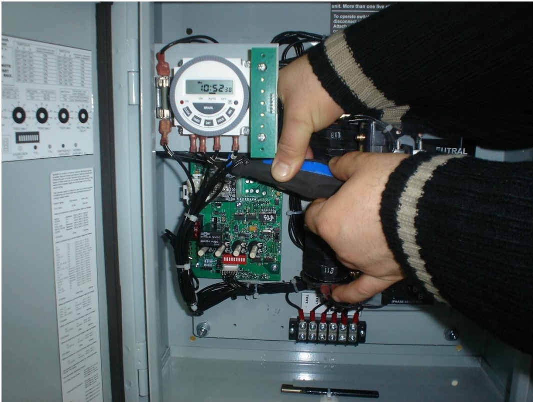
Figure 2. REMOVING THE TIMER SUPPORT BRACKET
