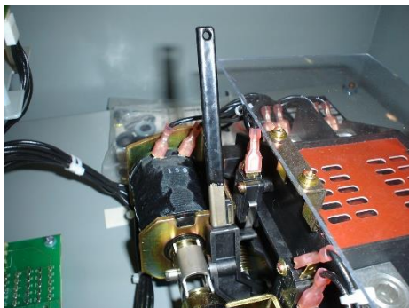
Manual transfer handle lever location
