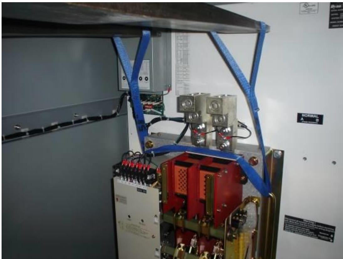
Figure 5. SWITCH REMOVAL
