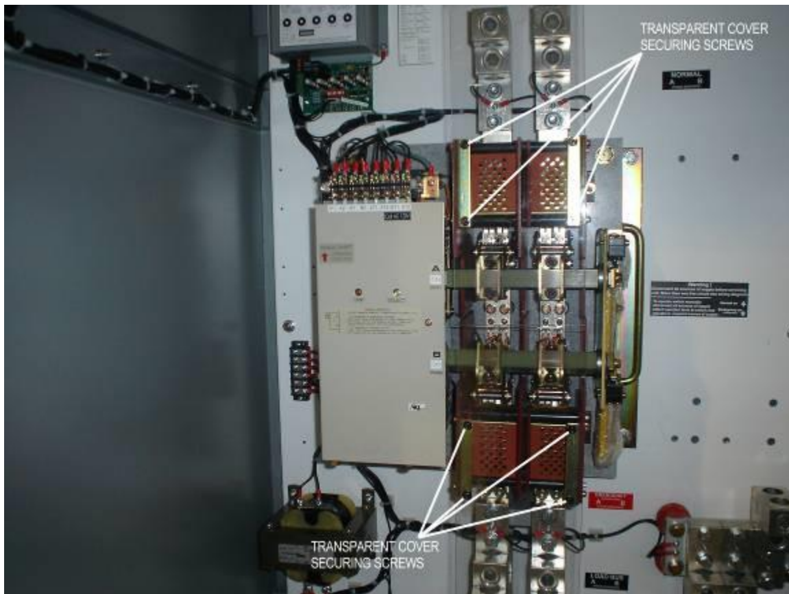
Figure 4. TRANSPARENT COVER SECURING SCREWS
