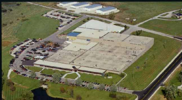
Generac's Waukesha facility • Wisconsin, USA
