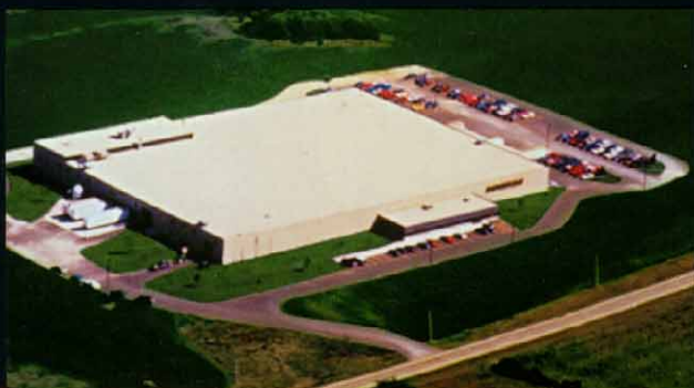
Generac's Whitewater facility • Wisconsin, USA
