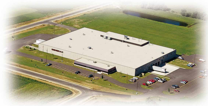
Eagle Facility - Eagle, Wisconsin
