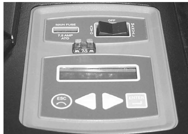
Figure 22. Remove 7.5 Amp Fuse
