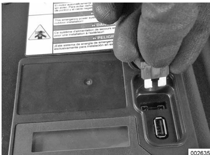
Figure 6-19. Remove 7.5 Amp Fuse
