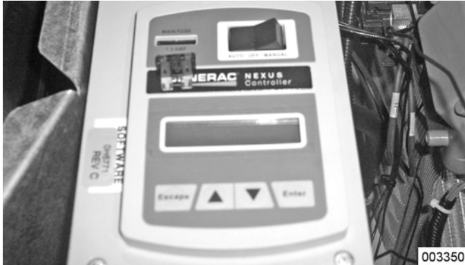
Figure 5-1. Remove 7.5 Amp Fuse (Nexus)
