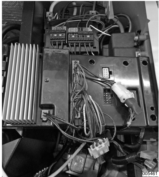
Figure 5-8. Evolution Controller Connections
