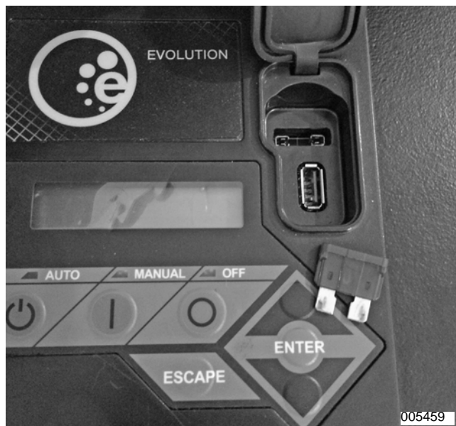
Figure 5-45. Remove 7.5 Amp Fuse (Evolution)
