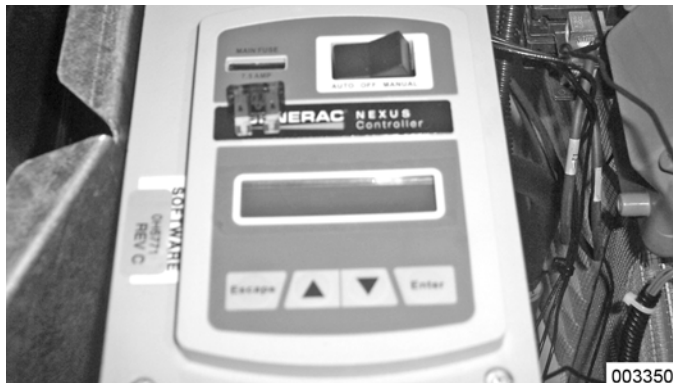
Figure 5-44. Remove 7.5 Amp Fuse (Nexus)
