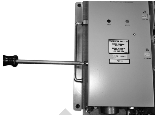
Figure 3. PCB Cover Removal
