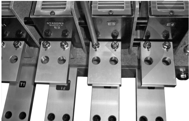
Figure 10. E1-E4 Lug Removal
