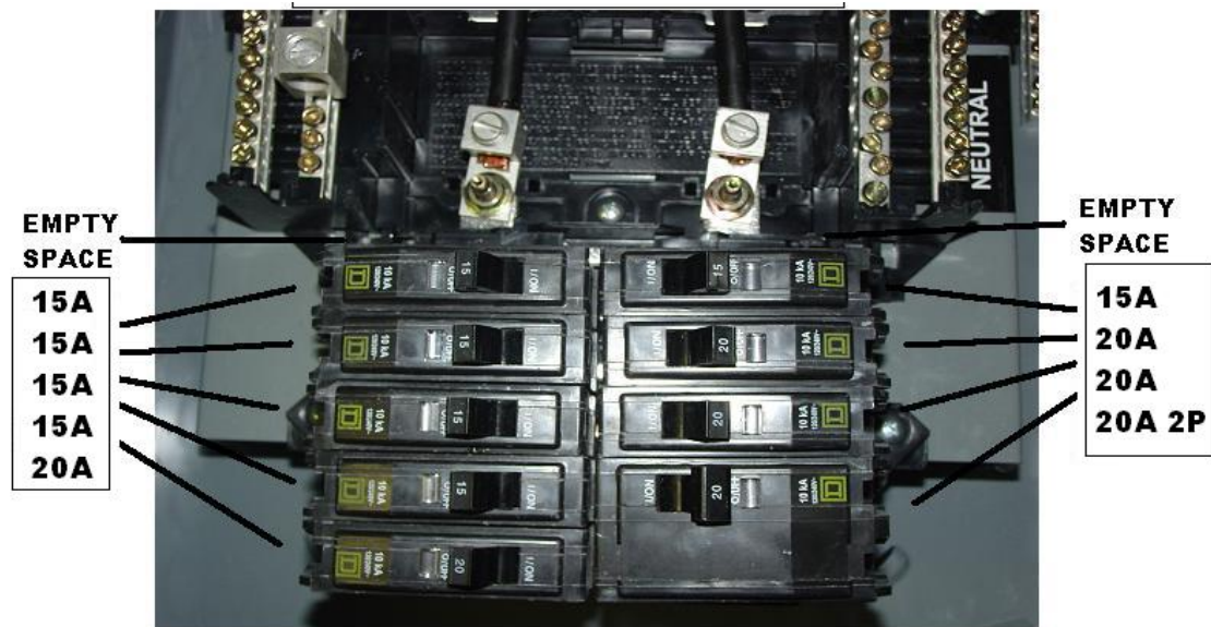
FIGURE 2: Standard Circuit Breaker Ratings/Locations
