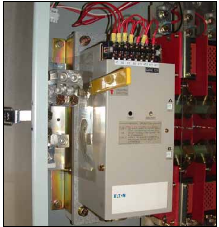
Figure 13. ATS Manual Operating Handle in Use.
