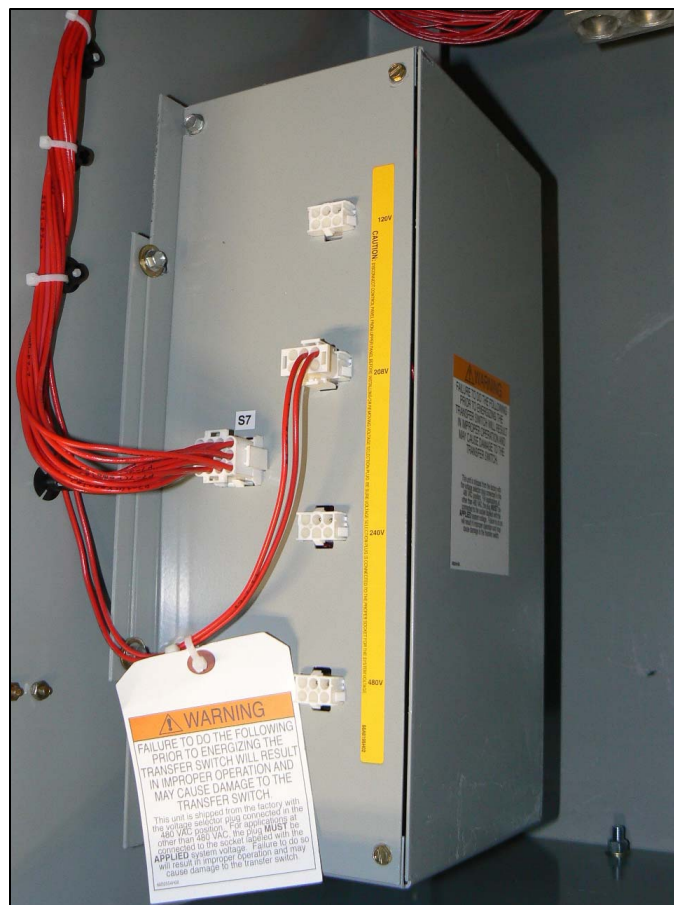
Figure 14. North American Market Voltage Selection Terminals (Shown Connected to the 208 Vac Plug).
