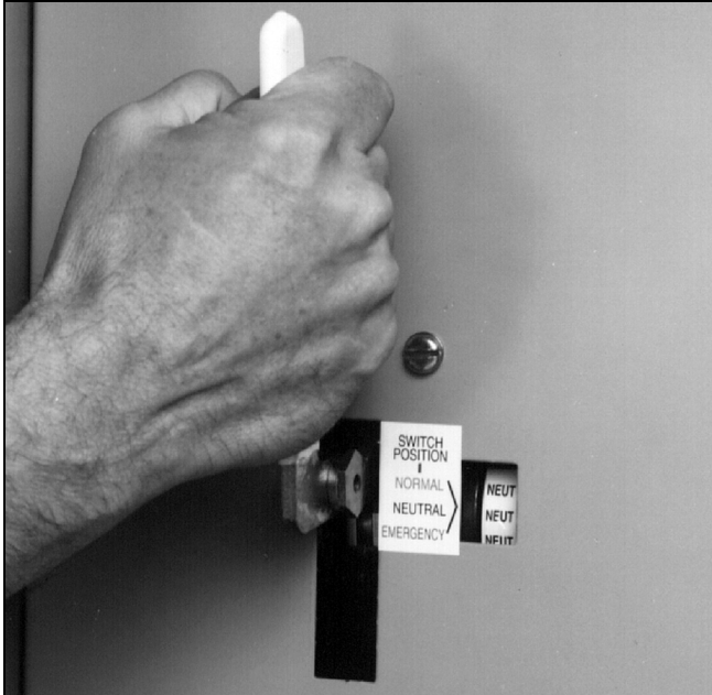
Figure 32.ATS Manual Operating Handle in Use (225-1200 A Models).
