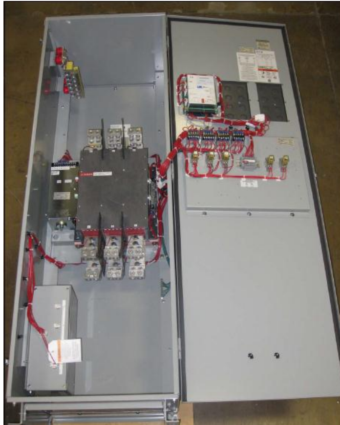
Typical Eaton Contactor ATS
