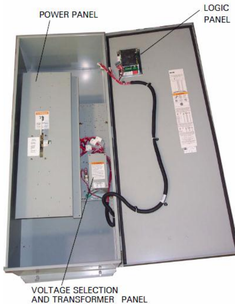
Typical Vertical Breaker Transfer Switch 225-600 Amps
