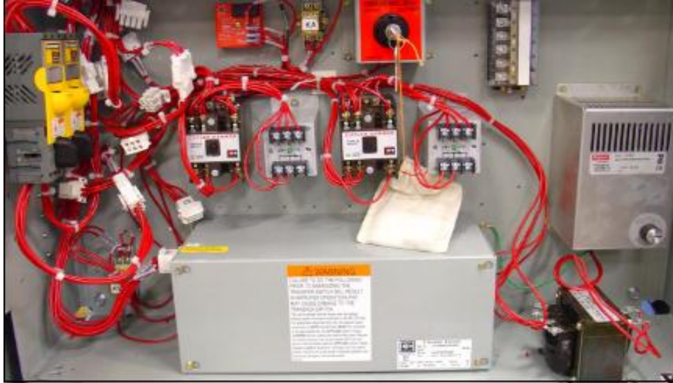
Transformer package in bottom of enclosure
