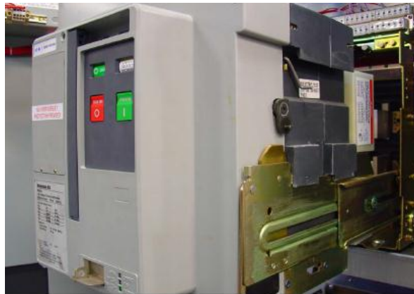
Drawout Switching Device
