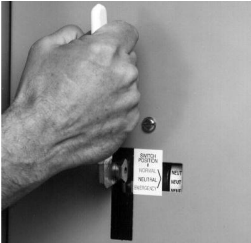
Typical 225 – 1000 Amp Manual Operation
