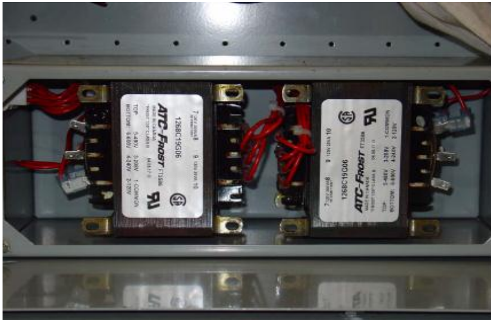
Transformer package in bottom of enclosure
