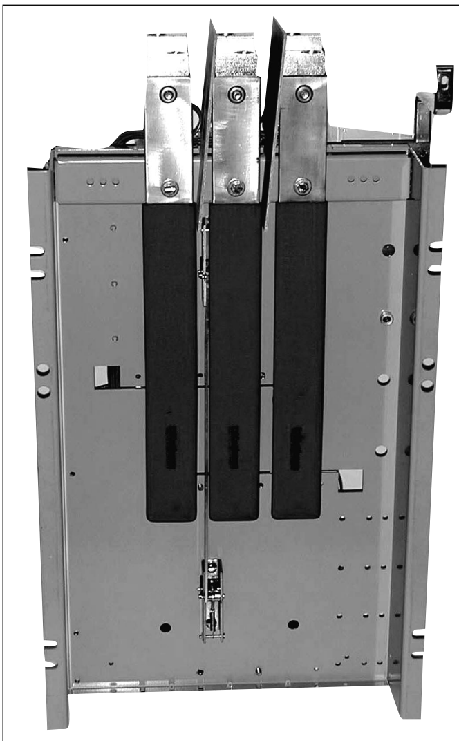
Figure 4-3 Mounted Load Lug Assembly (225-1000A Models)
