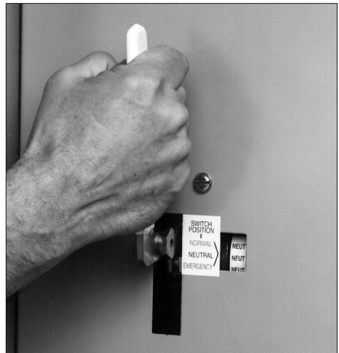
Figure 5-1 Transfer Switch Manual Operating Handle in Use (225-1000A Models)
