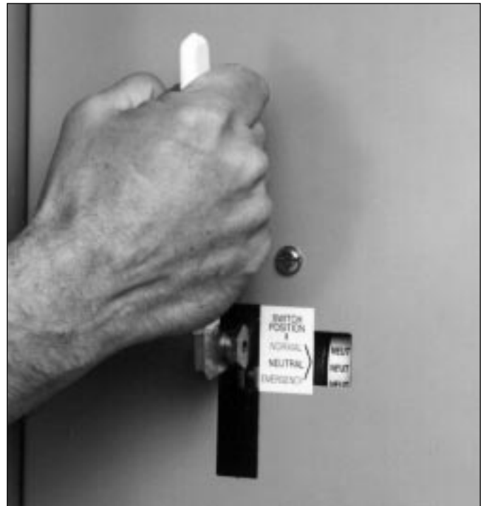
Figure 5-1 Transfer Switch Manual Operating Handle in Use (225-800A Models)
