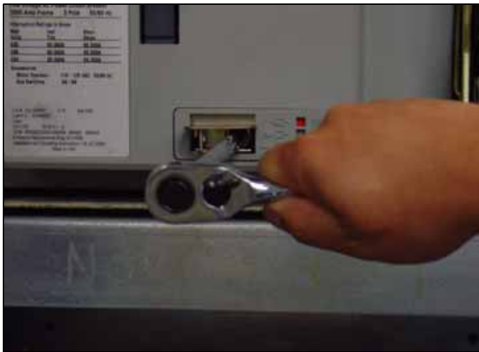
Figure 33. Levering and Position Indication.
