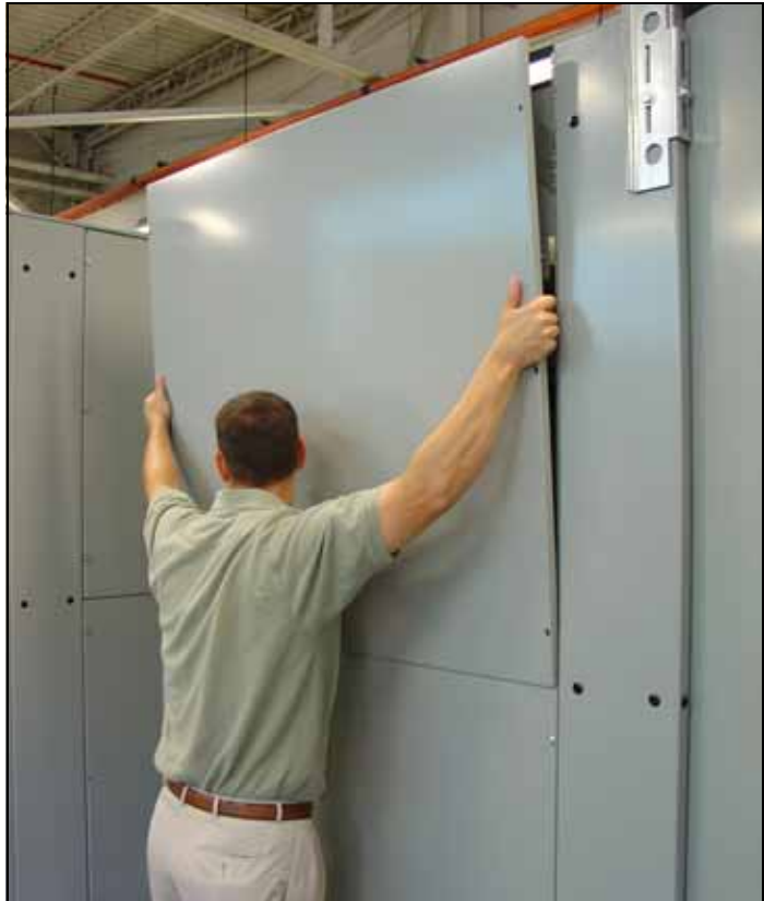
Figure 40. Tilting the Cover Away from the Frame.
