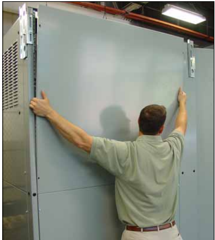
Figure 41. Lifting the Cover Free.
