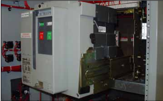
Figure 14. Drawout Mechanism (Closed Transition Shown)
