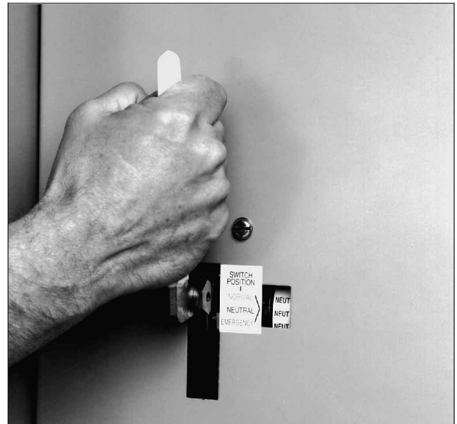
Figure 18. Transfer Switch Manual Operating Handle in Use on Vertical Design
