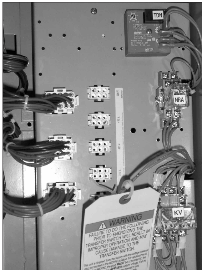
Figure 17. Line Voltage Plug and Receptacles (Shown with Covers Removed) for Horizontal Design
