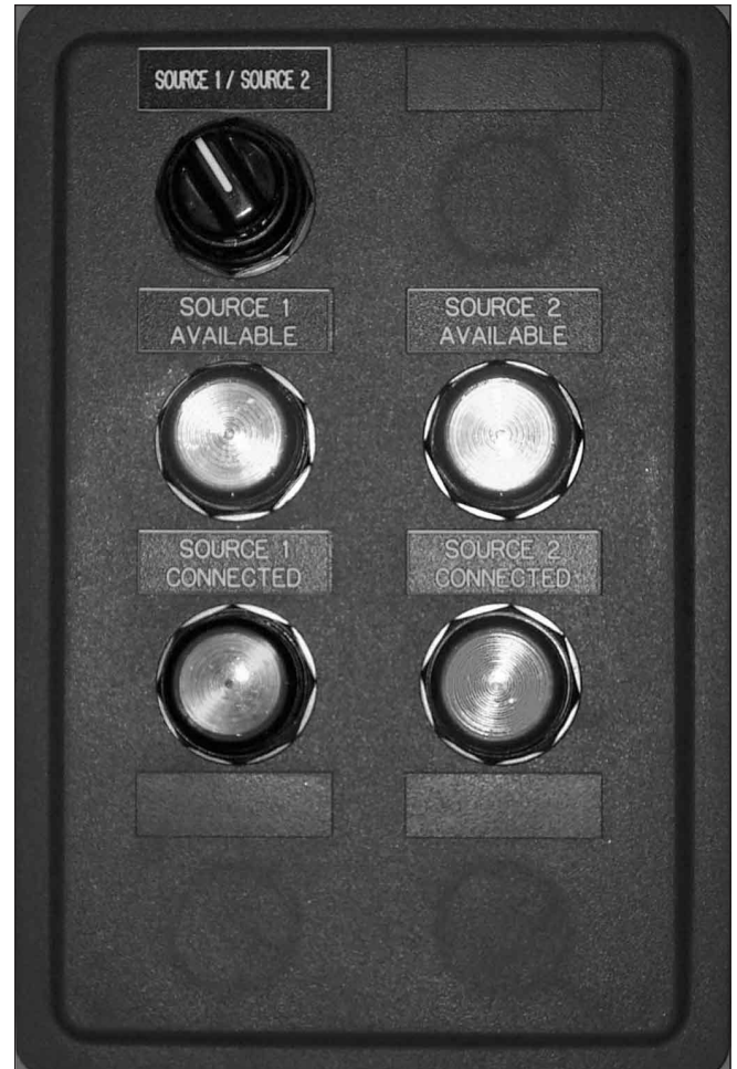
Figure 22. Electrical Operation Pushbutton and Position Indicating Lights Shown Mounted
