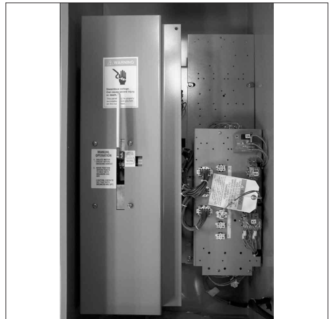
Figure 3. Vertical Design Automatic Transfer Switch Equipment with Deadfront Cover in Place Over Power Panel (225 – 1200 Amperes)
