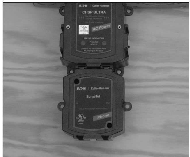
Figure 90. SurgeTel Mounted to the TVSS.
