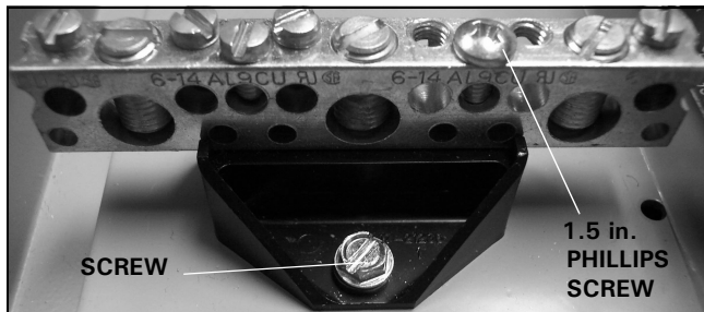
Figure 38. Replacing the Ground Bar.
