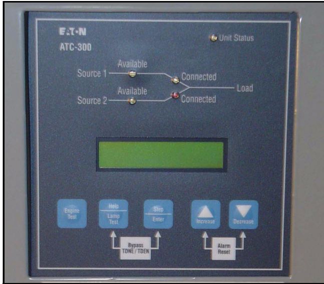
Figure 1. The ATC-300 Controller Front Panel.
