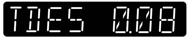
Figure 8. Typical Setpoints Display (Time Delay Engine Start - Minutes and Seconds).
