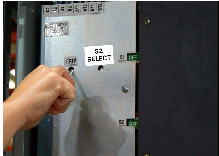
Figure 27. Manual Trip Location on the Mechanism.
