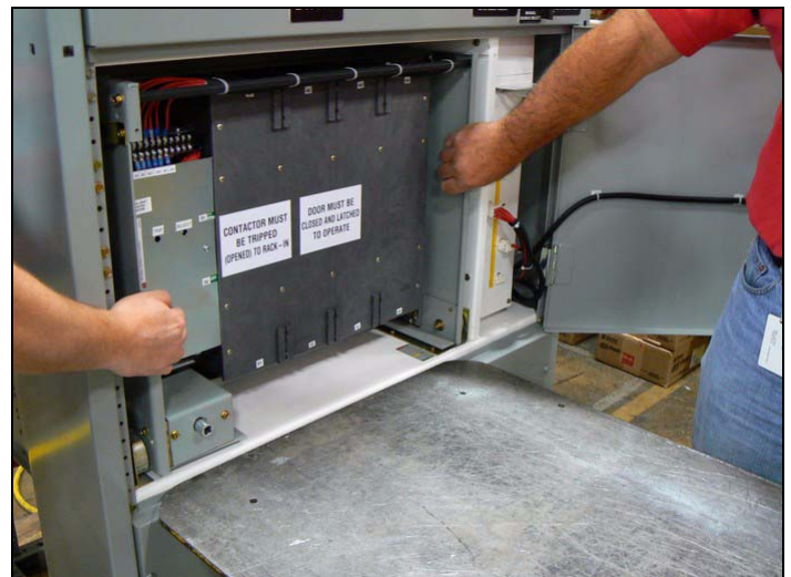
Figure 32. Removing the Lifting Mechanism.
