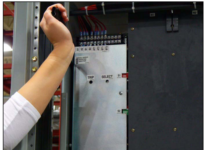
Figure 28. ATS Manual Operating Handle in Use.
