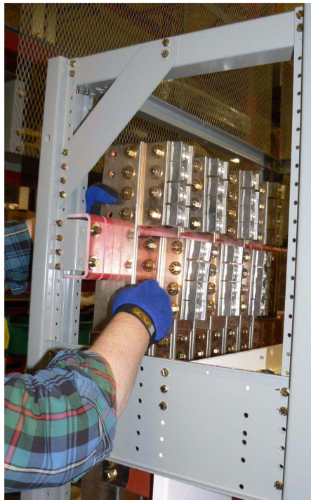
D. Reinstall Copper Extension.
