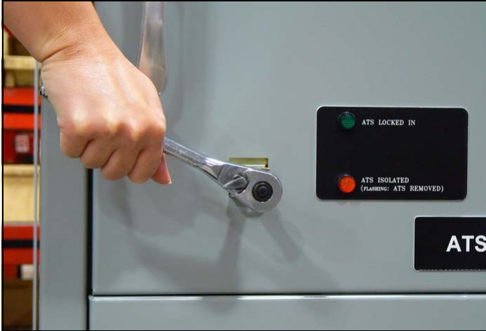
Figure 12. Draw-out Mechanism.
