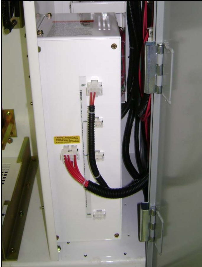
Figure 22. Voltage Selection Adjustment (120Vac is shown selected).
