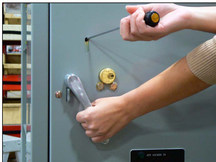
Figure 40. One must open the bottom door fist and then the Top door can be opened.
