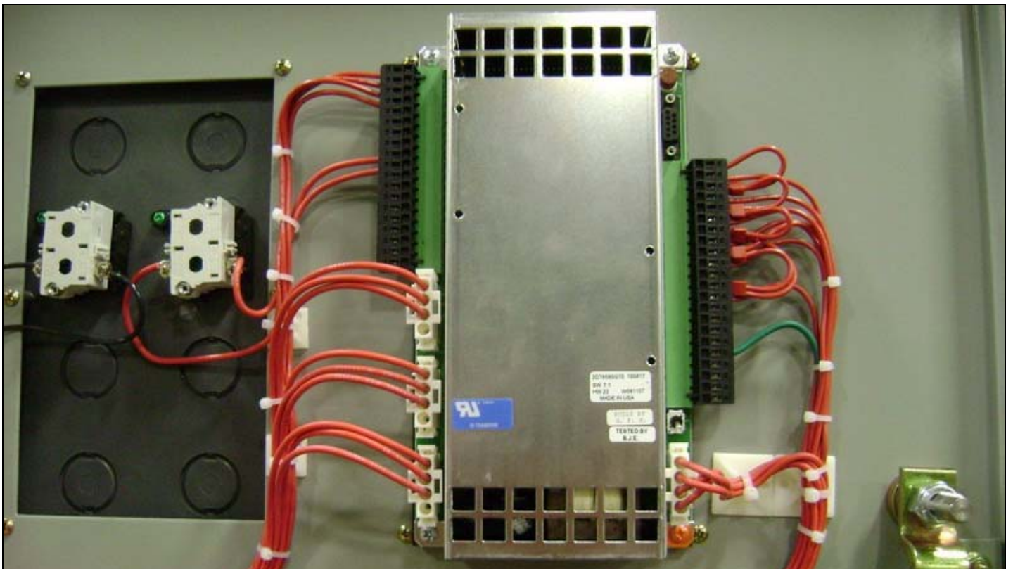
Figure 21B. Bypass Contactor ATS (Rear View of ATC-800 Controller).
