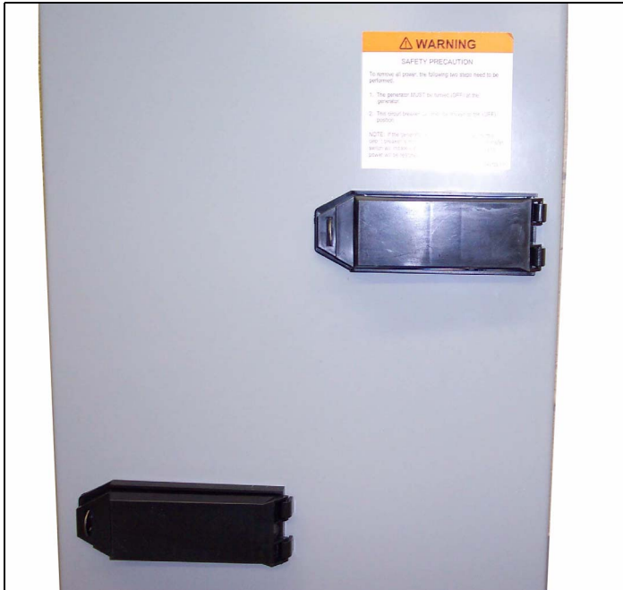
Figure 50. Service Entrance Cover Installed on the ATS Door.
