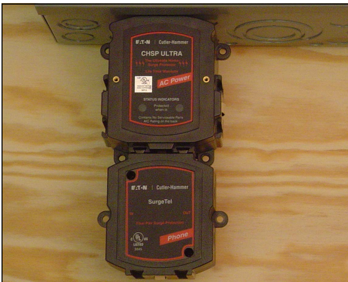
Figure 74. SurgeTel Mounted to the TVSS.
