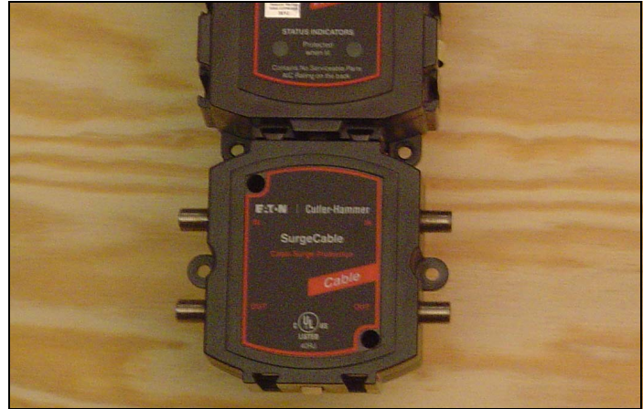
Figure 79. SurgeCable Mounted to the TVSS.
