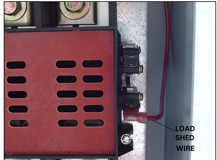
Figure 34. Optional Load Shed Wire Connected to the Auxiliary Switch on the Contactor.
