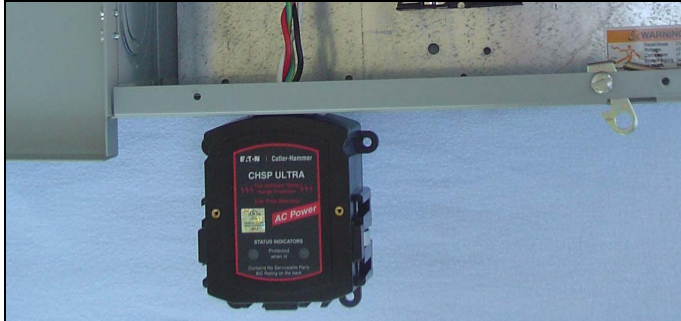
Figure 52. Possible Location for and Externally Mounted TVSS.
