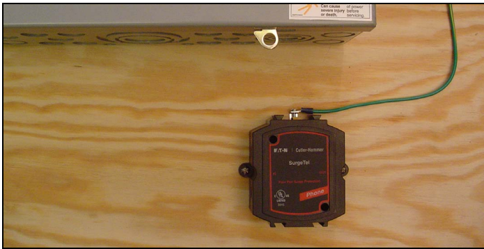
Figure 73. SurgeTel Mounted Externally When the TVSS Is Internally Mounted in a SE ATS.
