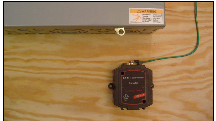
Figure 75. SurgeTel Installed Separate from the TVSS.
