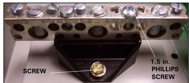
Figure 29. Replacing the Ground Bar.
