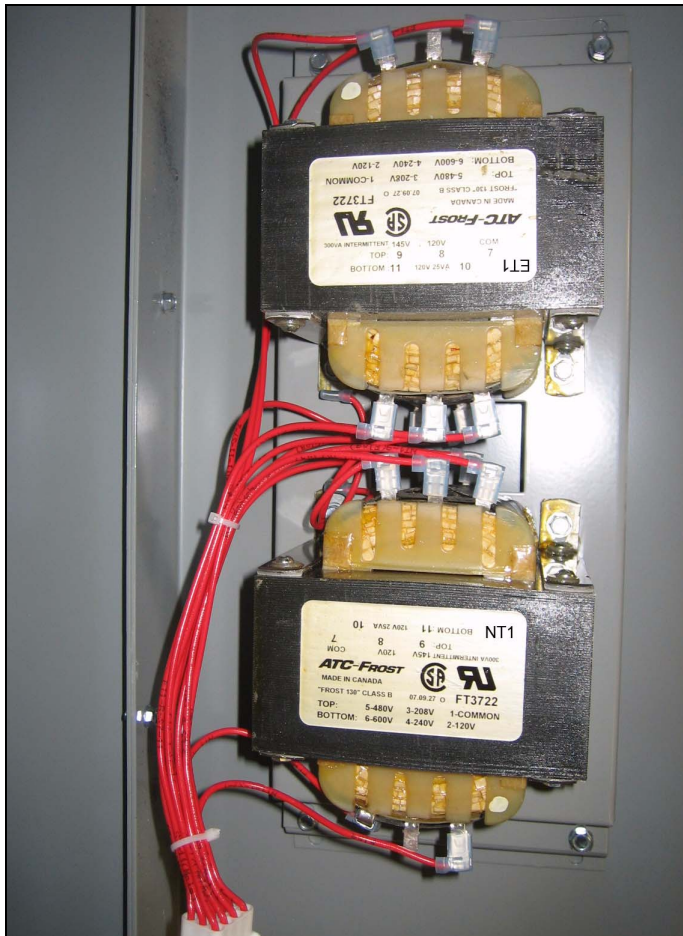
Figure 7. North American Market Voltage Selection Terminals (Shown Connected to the 480 Vac Taps).
