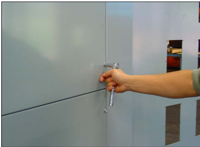
Figure 40. Removing the Bolts.
