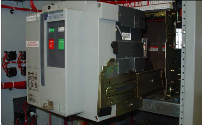
Figure 14. Drawout Mechanism (Closed Transition Shown)
