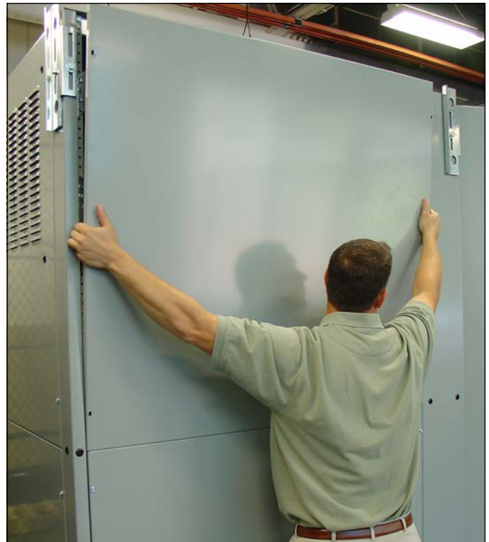
Figure 42. Lifting the Cover Free.
