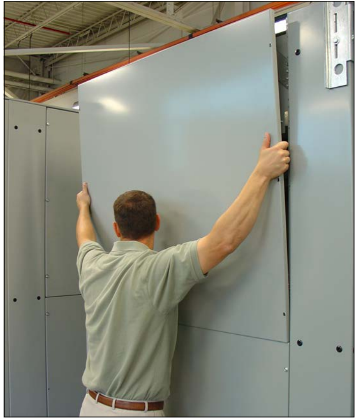
Figure 41. Tilting the Cover Away from the Frame.
