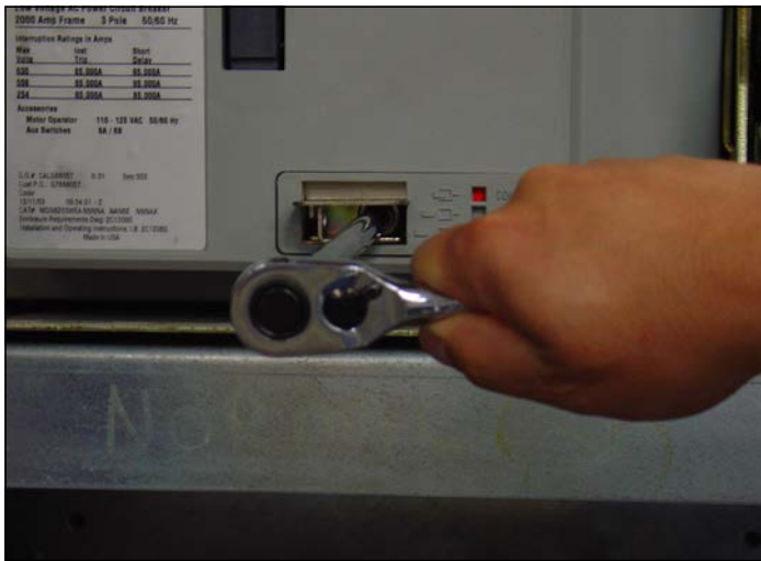
Figure 34. Levering and Position Indication.
