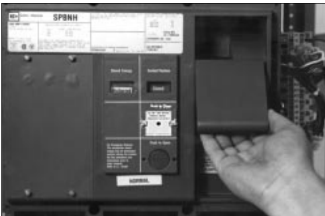
Figure 5-1 Pumping Handle Charges Stored Energy Mechanism
