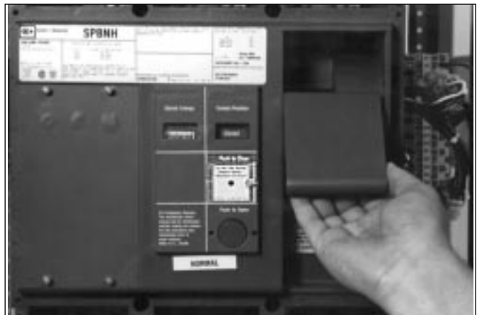
Figure 3-2 Insulated Case Switch
