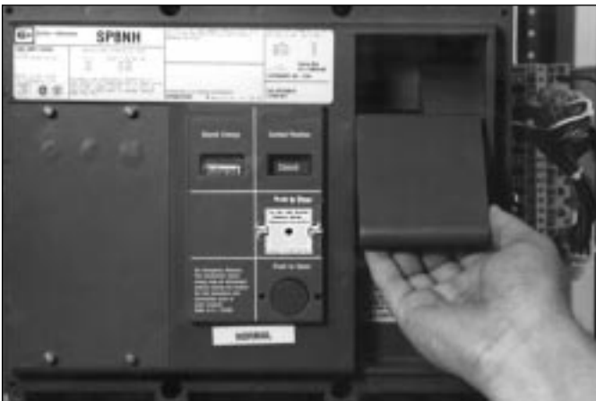
Figure 5-1 Pumping Handle Charges Stored Energy Mechanism
