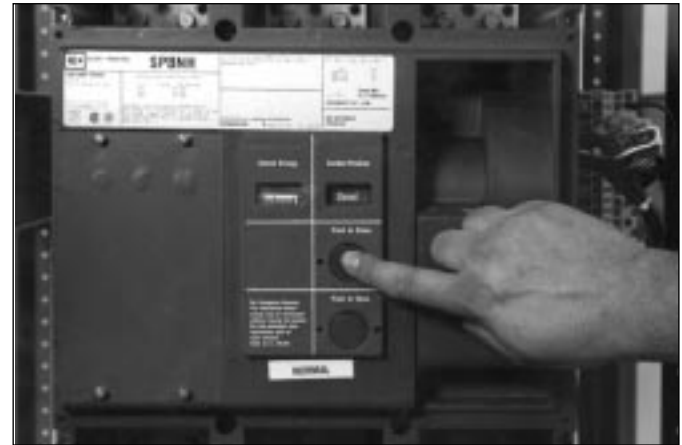
Figure 5-2 Close Switch by Pushing Close Button
