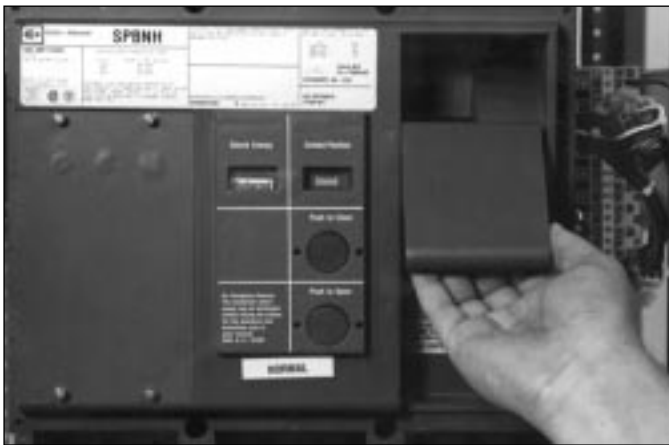
Figure 5-1 Pumping Handle Charges Stored Energy Mechanism
