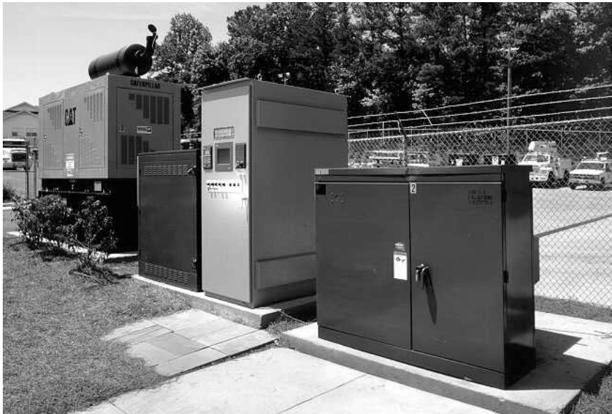
Figure 1. Peaking Switch installed with an existing transfer switch to provide full-time paralleling capability.
