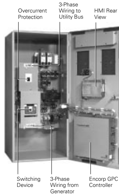
540A Peaking Switch — Interior View
