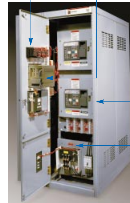
Drawout SPB Insulated Case Switches or Circuit Breakers
