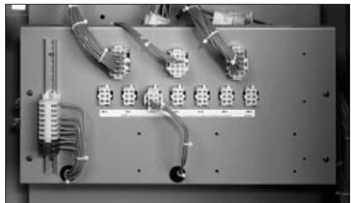
Figure 4-6 Line Voltage Plug and Receptacles (shown with covers removed) for Horizontal Design
