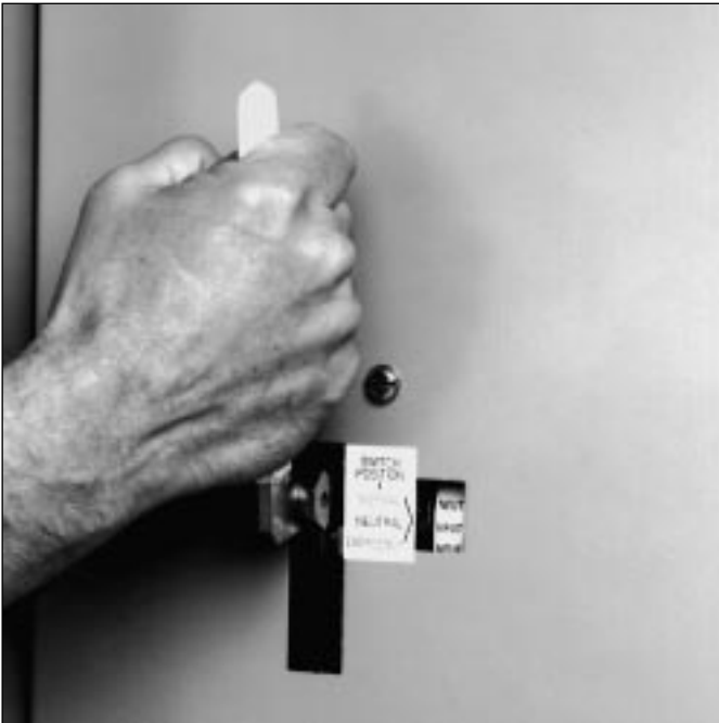
Figure 5-1 Transfer Switch Manual Operating Handle in Use on Vertical Design
