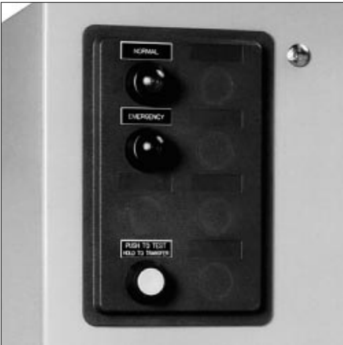
Figure 5-5 Electrical Operation Pushbutton and Position Indicating Lights Shown Mounted
