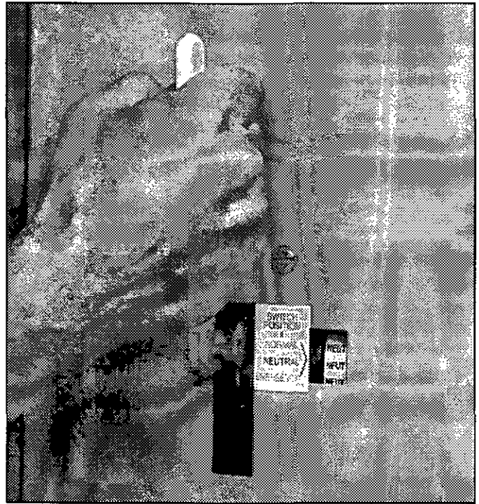
Figure 5-1 Transfer Switch Manual Operating Handle in Use (300-600A Models)
