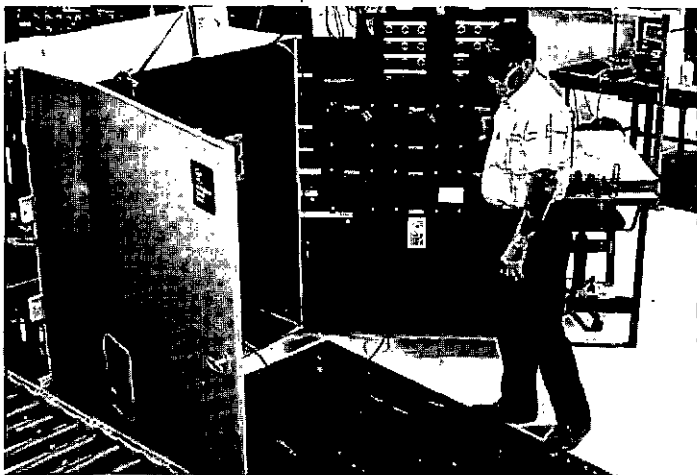
Units are cycled 50 times by alternately removing normal and emergency power sources.
